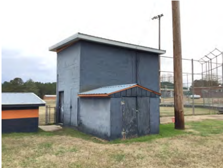
1). North Elevation - Feb 06, 2017
