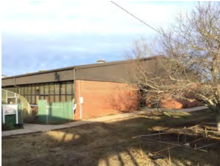
4). Southeast Elevation - Feb 12, 2017
