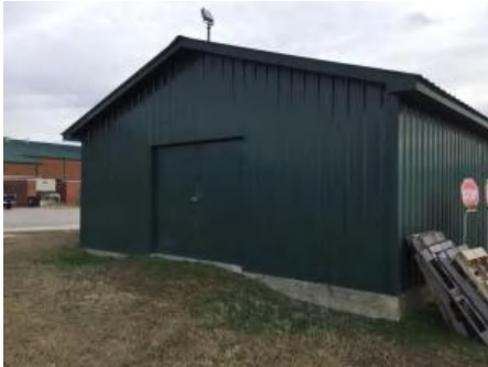
1). North Elevation - Jan 12, 2017
