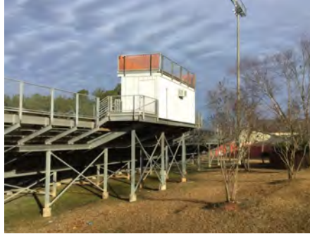
2). Southeast Elevation - Feb 12, 2017
