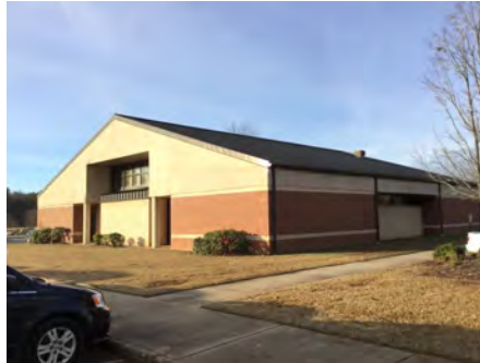
2). Northeast Elevation - Feb 12, 2017
