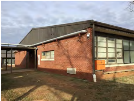
4). South Elevation - Feb 12, 2017
