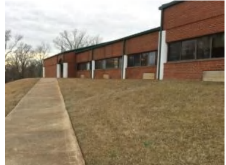
3). Southeast Elevation - Mar 06, 2017
