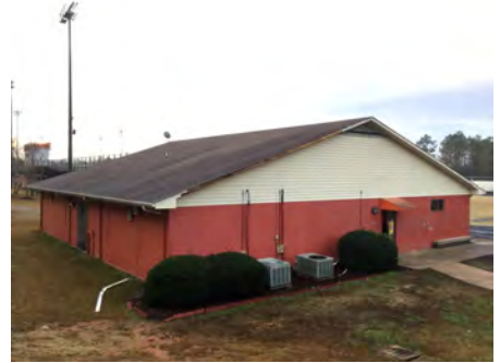
3). North Elevation - Feb 12, 2017
