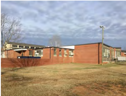
4). Southeast Elevation - Feb 16, 2017
