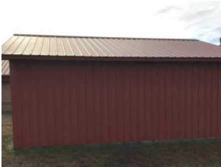
4). North Elevation - Mar 07, 2017
