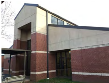
2). North Elevation - Feb 16, 2017
