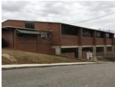
2). Southwest Elevation - Jan 20, 2017
