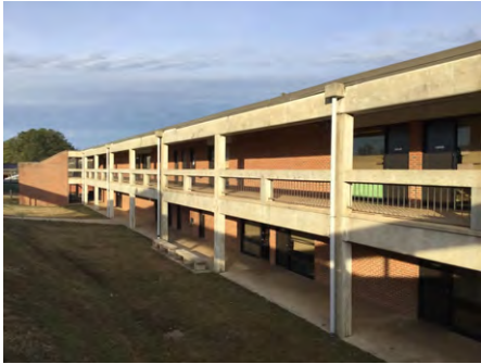
1). South Elevation - Feb 12, 2017
