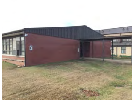
2). North Elevation - Feb 12, 2017
