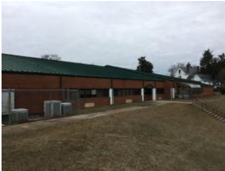
4). East Elevation - Mar 06, 2017
