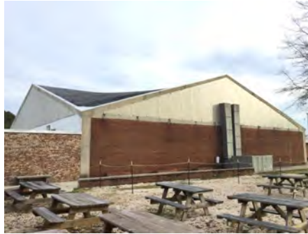
2). South Elevation - Feb 06, 2017
