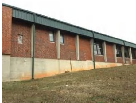
2). Southeast Elevation - Feb 10, 2017
