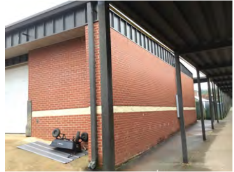
3). South Elevation - Feb 12, 2017
