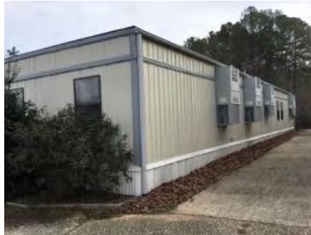
2). Northwest Elevation - Jan 19, 2017
