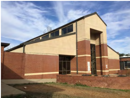
1). South Elevation - Feb 16, 2017
