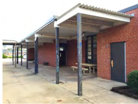
2). North Elevation - Feb 16, 2017
