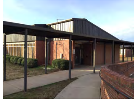
3). North Elevation - Feb 12, 2017
