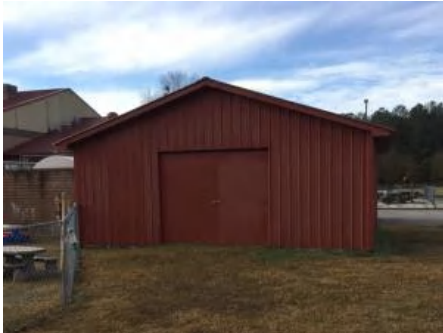
1). East Elevation - Mar 07, 2017
