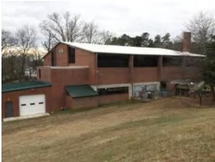
4). Northeast Elevation - Feb 09, 2017
