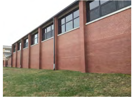
3). South Elevation - Feb 16, 2017
