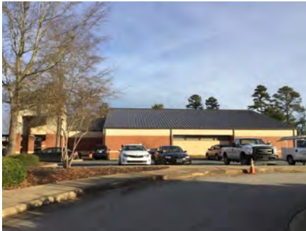
4). South Elevation - Feb 12, 2017
