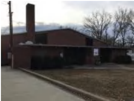
1). Northwest Elevation - Jan 20, 2017
