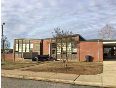
1). East Elevation - Feb 16, 2017
