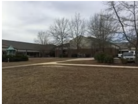
2). North Elevation - Feb 08, 2017
