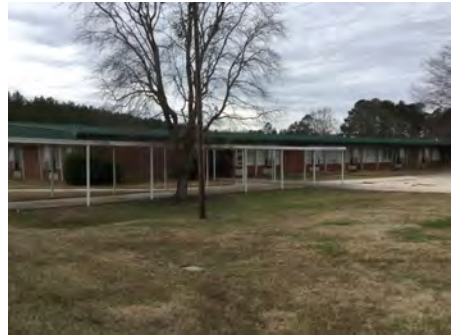
6). Northeast Elevation - Feb 06, 2017
