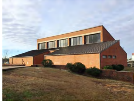
2). Northeast Elevation - Feb 16, 2017
