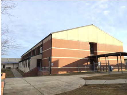
1). South Elevation - Feb 12, 2017
