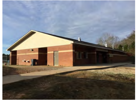
3). Northeast Elevation - Feb 12, 2017
