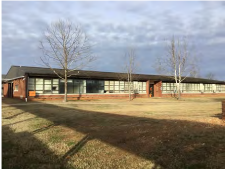
1). East Elevation - Feb 12, 2017
