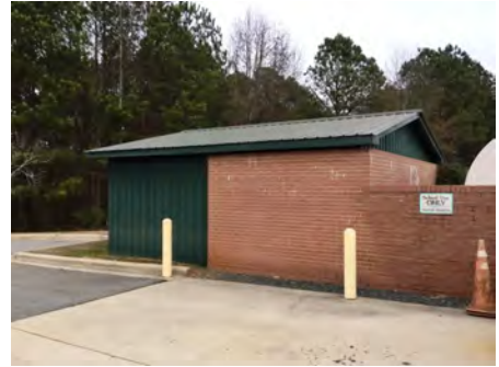
3). Southwest Elevation - Jan 19, 2017
