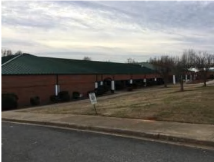
1). Northwest Elevation - Mar 06, 2017
