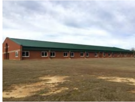
2). Southeast Elevation - Feb 08, 2017
