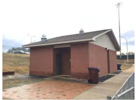
3). North Elevation - Feb 12, 2017
