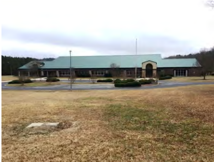
1). North Elevation - Jan 19, 2017
