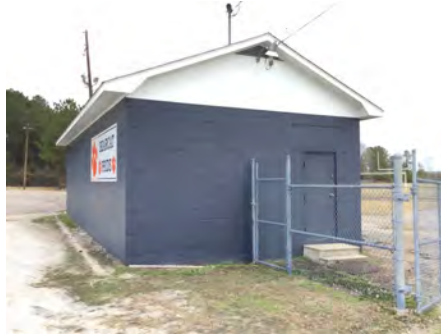
2). South Elevation - Feb 06, 2017
