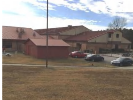
2). North Elevation - Jan 09, 2017
