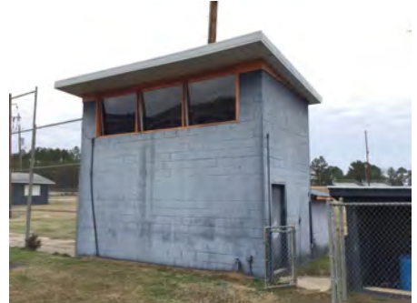
3). South Elevation - Feb 06, 2017
