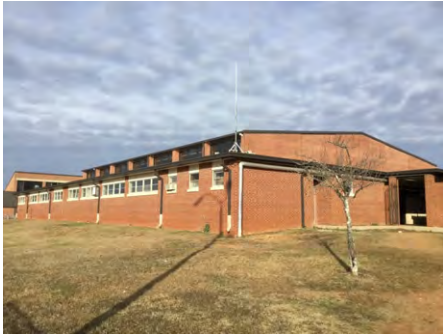
1). Southeast Elevation - Feb 16, 2017
