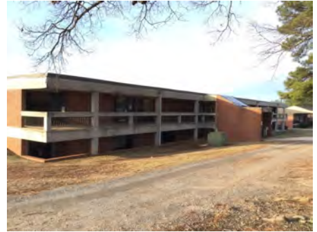
3). North Elevation - Feb 12, 2017
