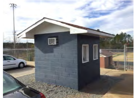
3). Northeast Elevation - Feb 15, 2017
