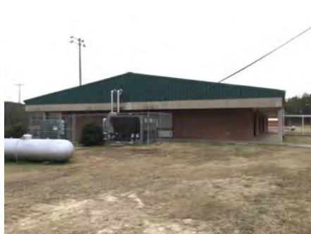
2). North Elevation - Feb 06, 2017
