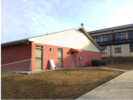
1). South Elevation - Feb 12, 2017
