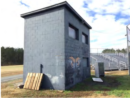
1). Northeast Elevation - Feb 15, 2017
