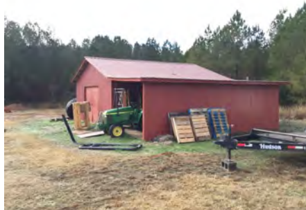
2). North Elevation - Feb 12, 2017
