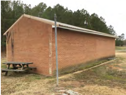
4). Northeast Elevation - Feb 06, 2017
