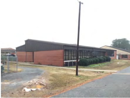
1). Northeast Elevation - Feb 12, 2017
