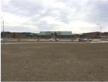
1). Northeast Elevation - Feb 08, 2017
