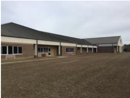
4). South Elevation - Feb 08, 2017
