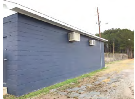
3). East Elevation - Feb 06, 2017
