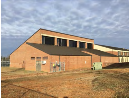
1). Southeast Elevation - Feb 16, 2017
