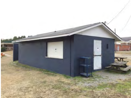
1). Northeast Elevation - Feb 06, 2017
