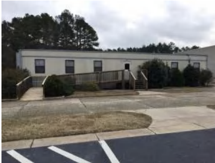
1). North Elevation - Jan 19, 2017
