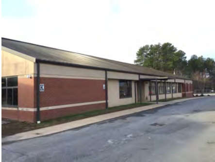
4). North Elevation - Feb 12, 2017
