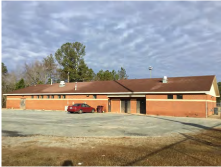
1). South Elevation - Feb 12, 2017
