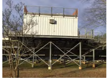
3). South Elevation - Feb 12, 2017
