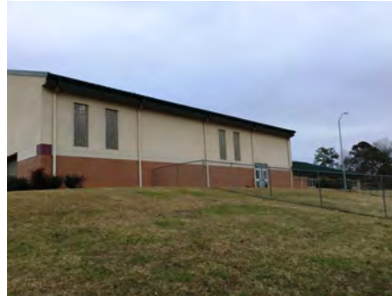
2). Southwest Elevation - Jan 19, 2017
