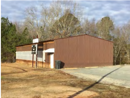
1). Southeast Elevation - Feb 15, 2017
