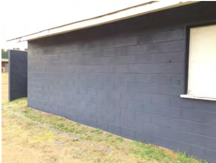
4). East Elevation - Feb 06, 2017
